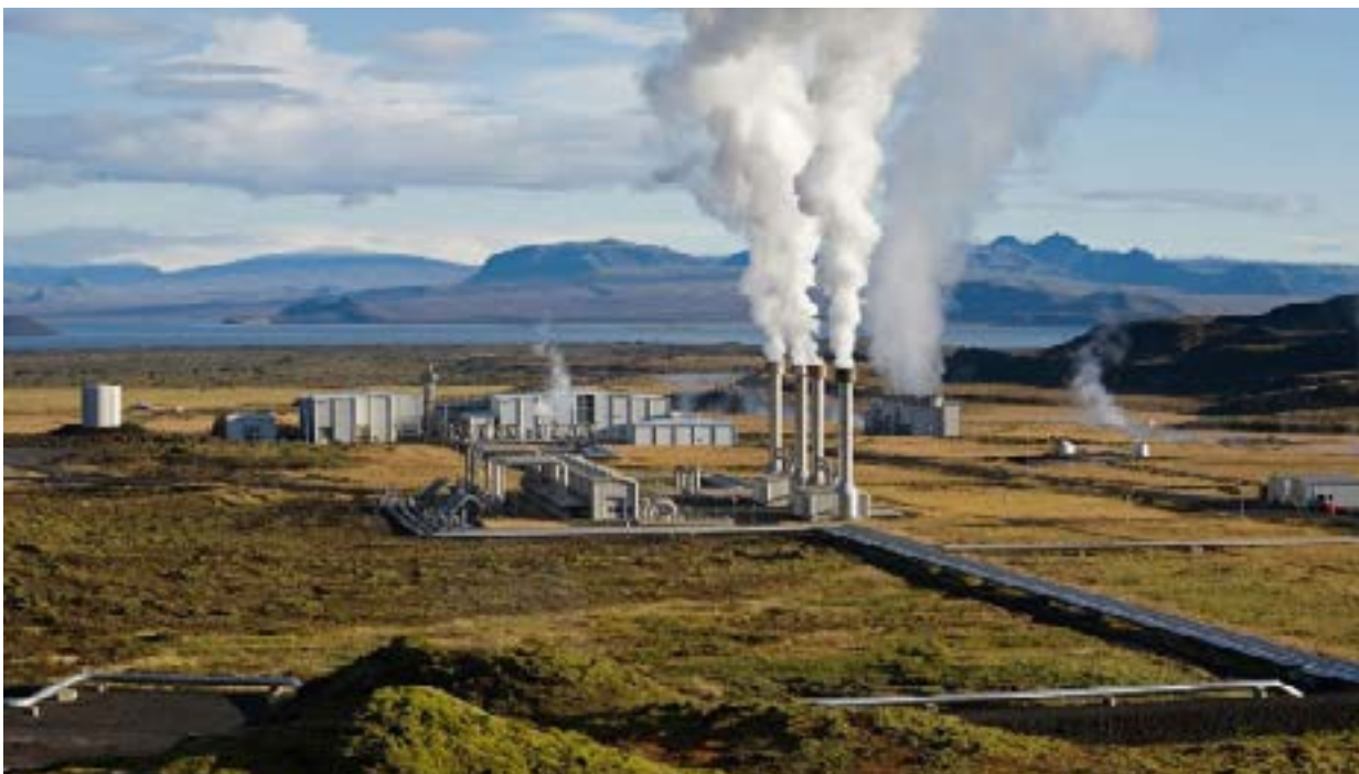
Figure (12): One of the geothermal energy production stations
